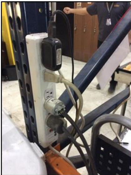
(Power strips permanently mounted / daisy chained)
